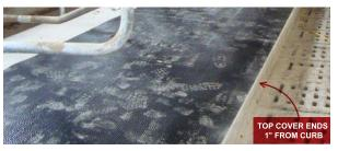
by a cow. If additional anchors are required to hold down the mattress cover on the curb end, 2" anchors should be placed as needed.
